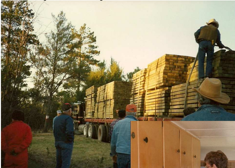
1987 rebuilding the Luzerne Bridge
